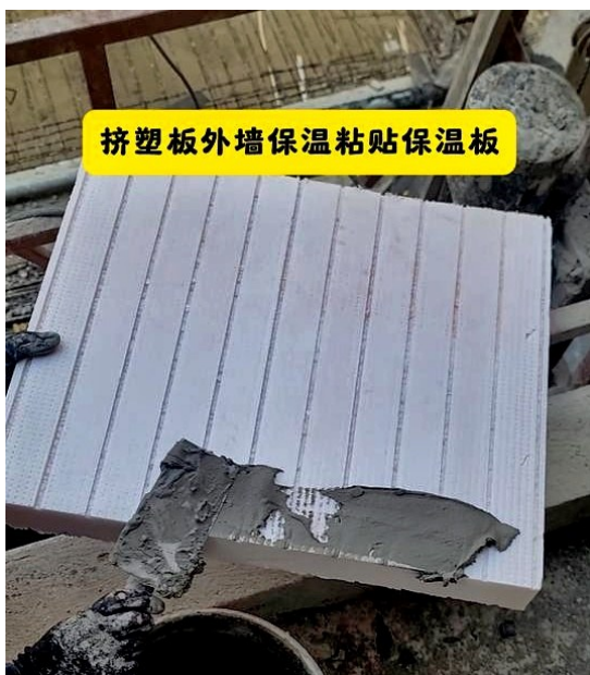
图3 粘贴挤塑板技术实景示意图(图片来源: https://mbd.baidu.com/newspage/data/videolanding?nid=sv_4097503392333269316&sourceFrom=qmj )
